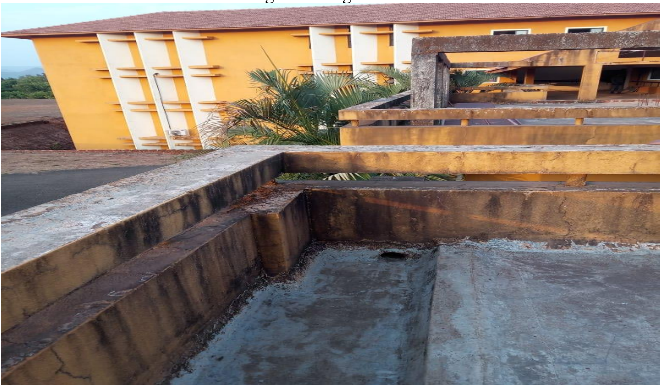
Water routing towards ground from roof
