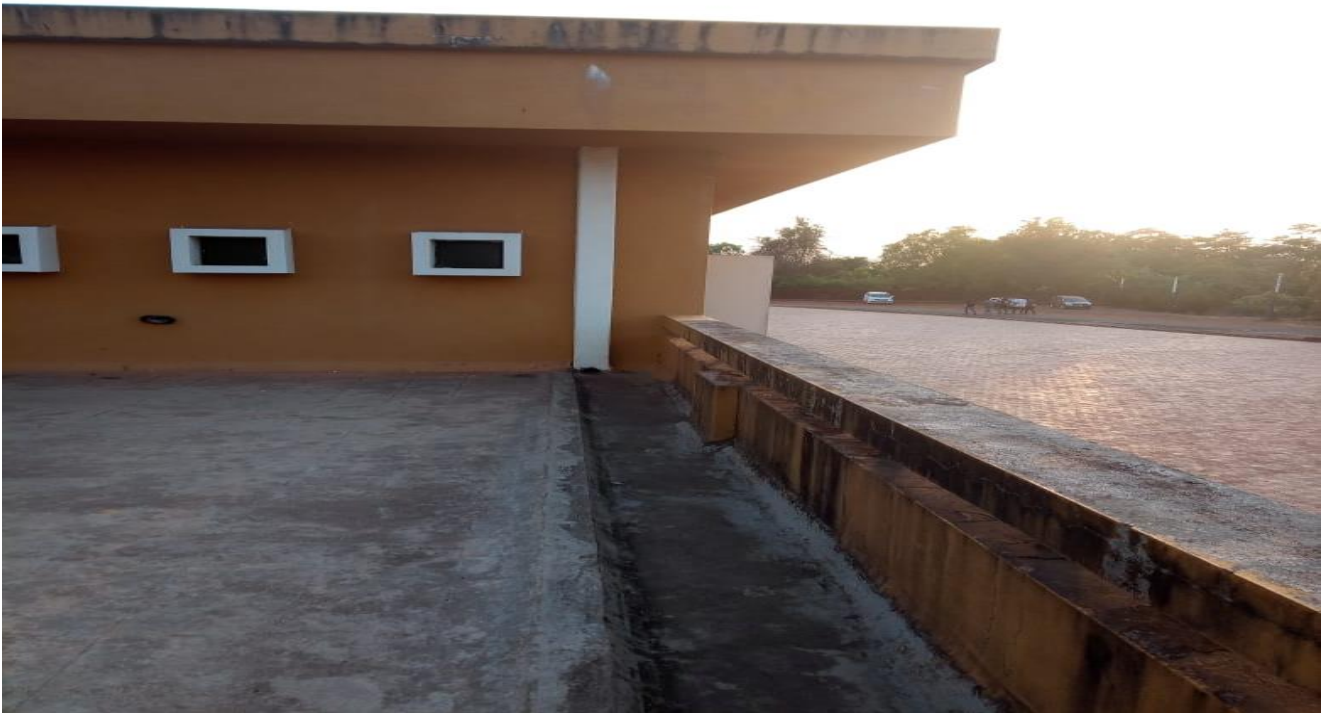
Water routing towards ground from roof
