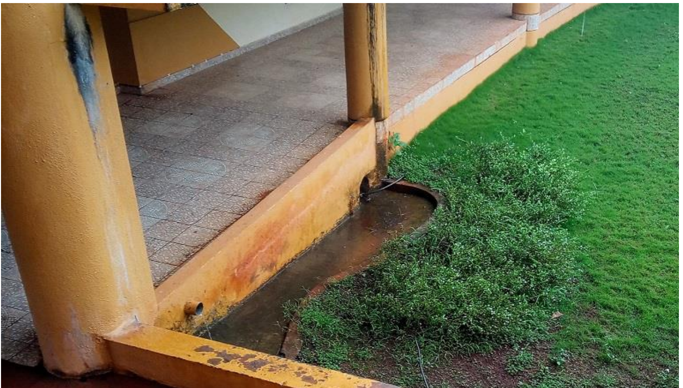
Rain Water routing near office
