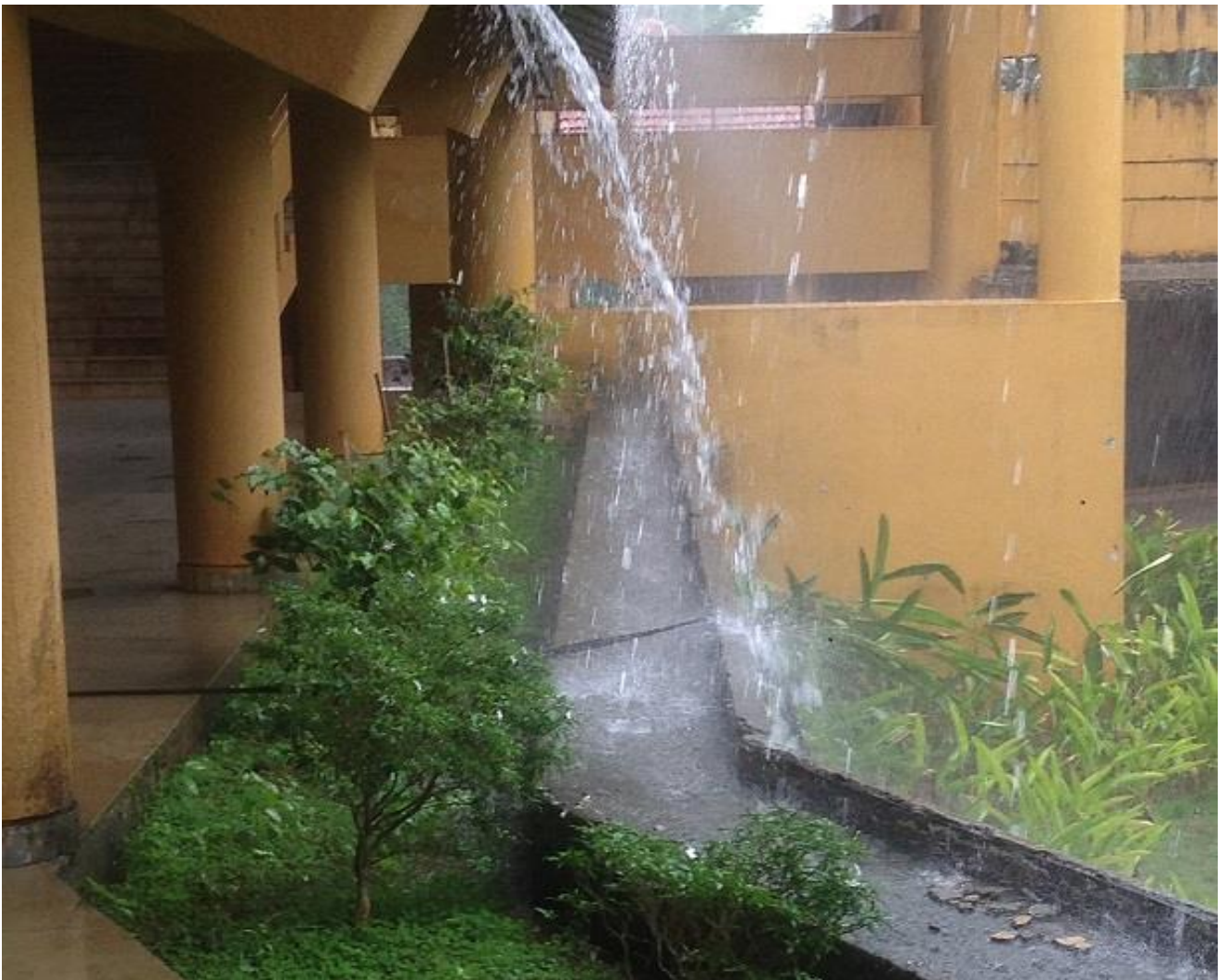
Water harvesting in corridor
